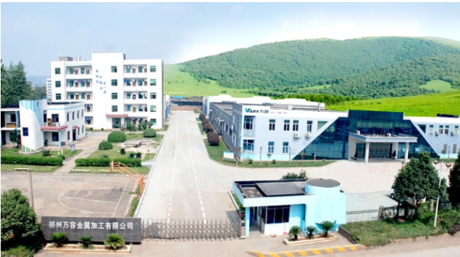
Chenzhou Operation Base
